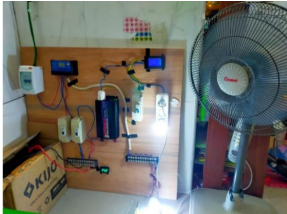
Fig 3. The results of making 240 WP offgrid PLTS rooftop residential houses have successfully turned on with DC output (DC lights) and AC output (AC lights and fans)
