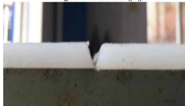
Figure 3. Preparation of the V-Groove
